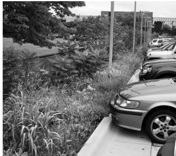
Bioswales slow, cleanse, and cool surplus rainwater on site.
